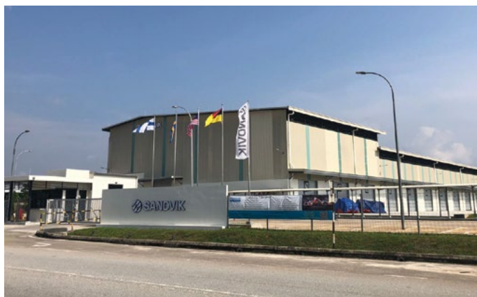
Axis Industrial Facility @ Sendayan
