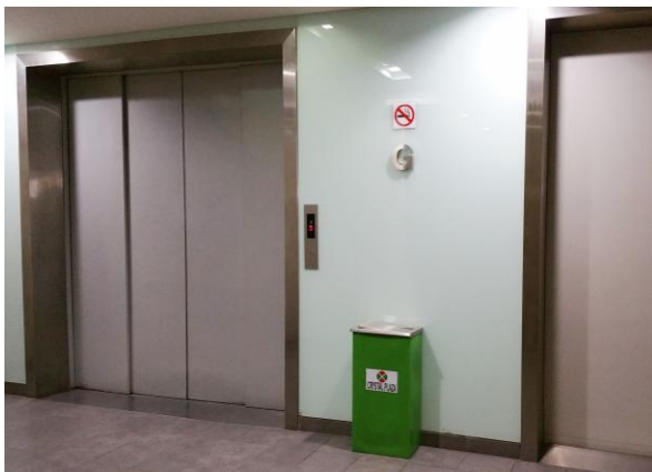
Cargo Lift Lobby
