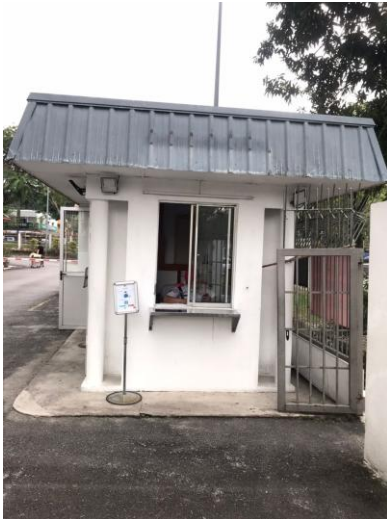
Entrance Guard Post
