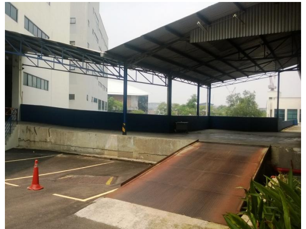
Loading area with 2 loading bays
