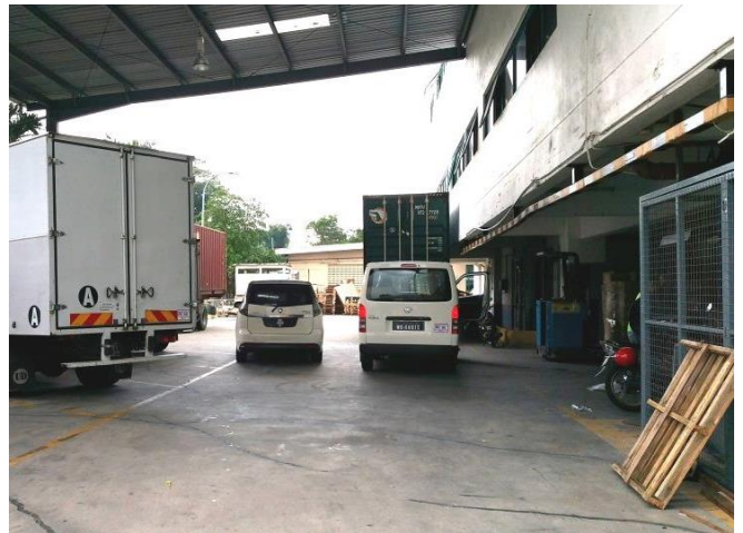
Loading/ Unloading Bay Docks
