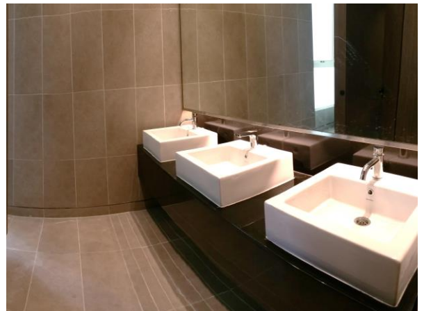
Newly Refurbished Toilets
