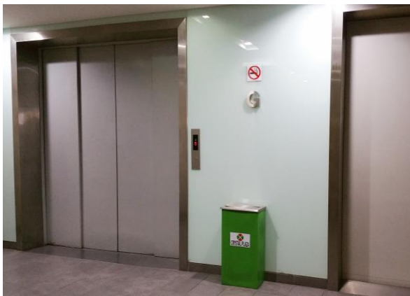
Cargo Lift Lobby
