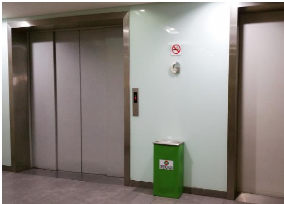
Cargo Lift Lobby
