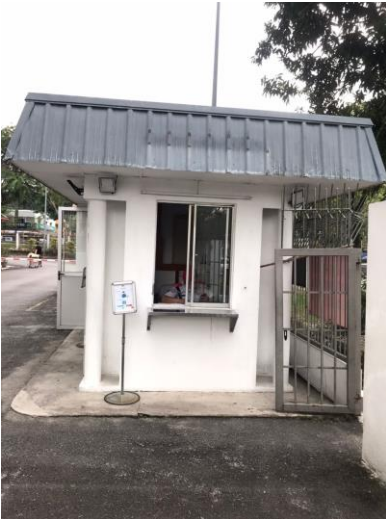
Entrance Guard Post
