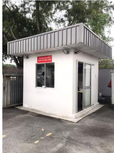
Exit Guard Post
