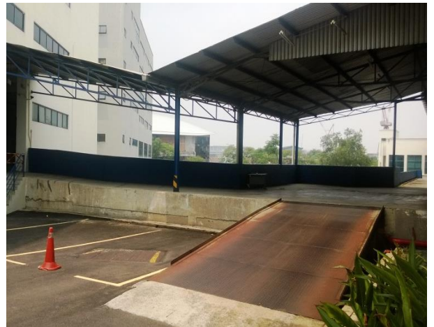
Loading area with 2 loading bays
