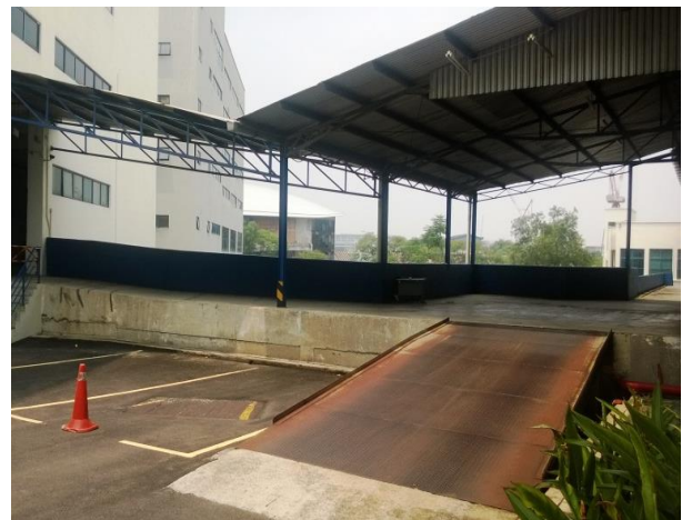
Loading area with 2 loading bays
