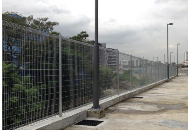
Anti Climb Perimeter Fencing
